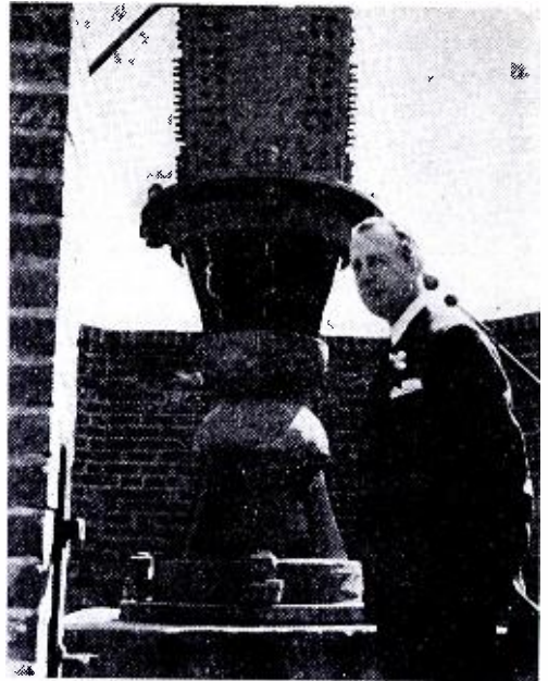
Mr. Powel Crosley, Jr., standing at the base of the 831-ft. vertical antenna tower of WLW at Cincinnati. A load of more than 900,000 pounds rests on the seemingly fragile porcelain insulator base. The two porcelain pieces are cup-like in shape with walls less than two inches thick. This antenna rises 250 feet higher than the Washington Monument.
